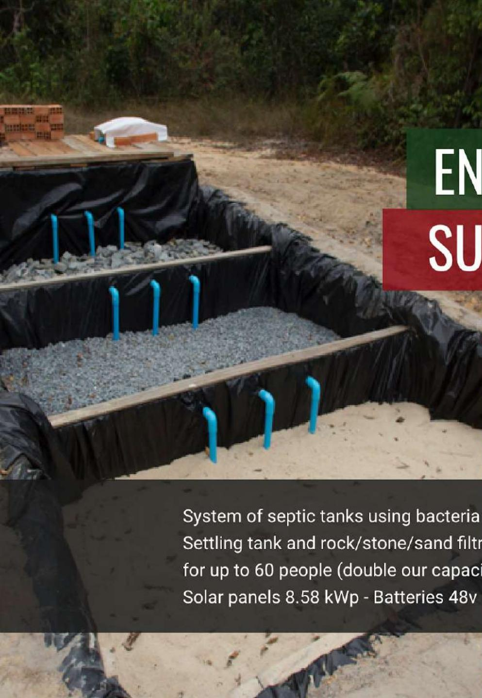
System of septic tanks using bacteria for solid waste.
